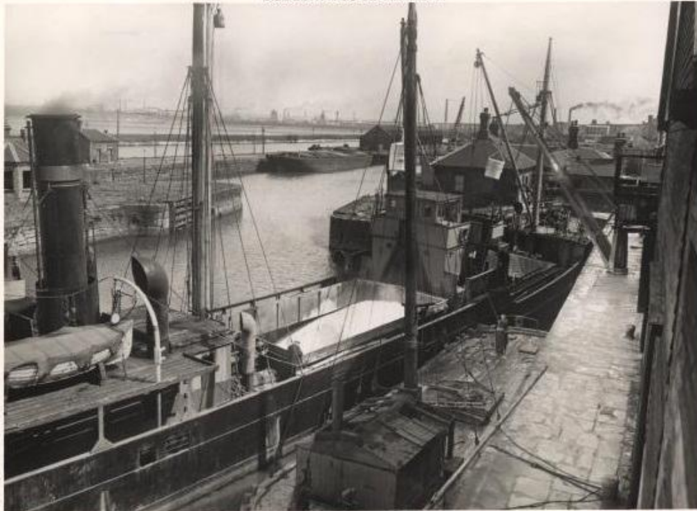
RUNCORN DOCKS Cargo of China Clay in process of discharge Ex S.S. "MOELFRE ROSE" to the Alfred Dock Sheds
